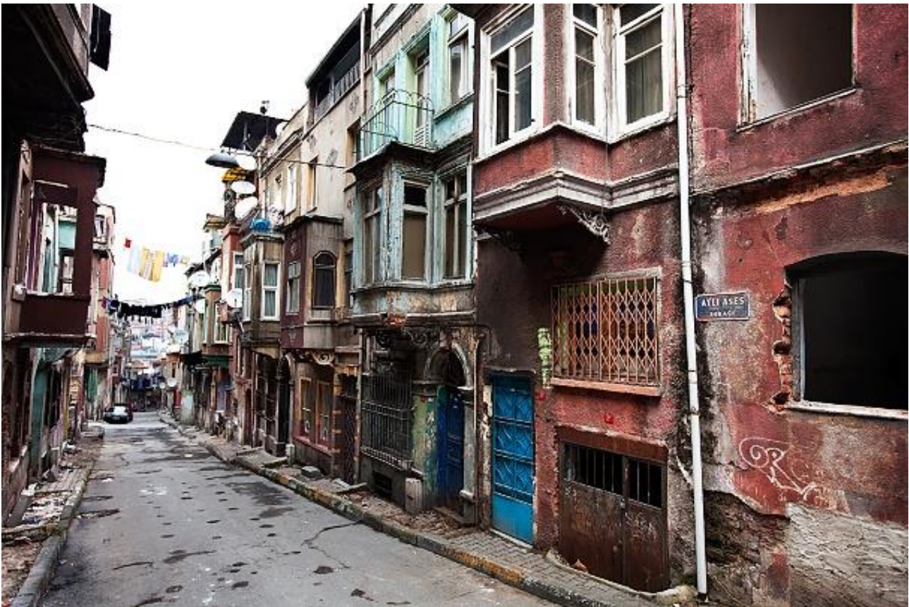
Fig. 1 Abandoned buildings in Tarlabası, İstanbul [2].
