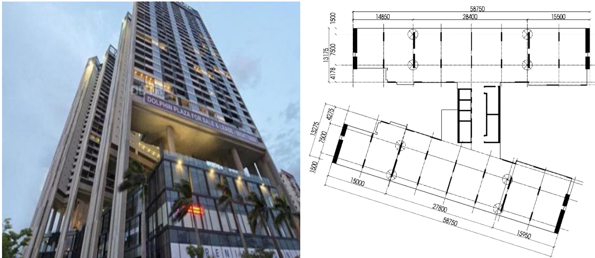
Fig. 1 a) Image of the building; b) Layout of transferred structure.
