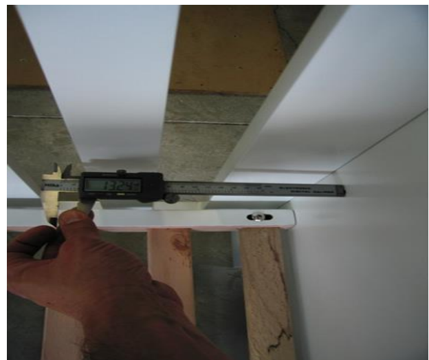
Fig. 1 Measurement of the assembling holes.
