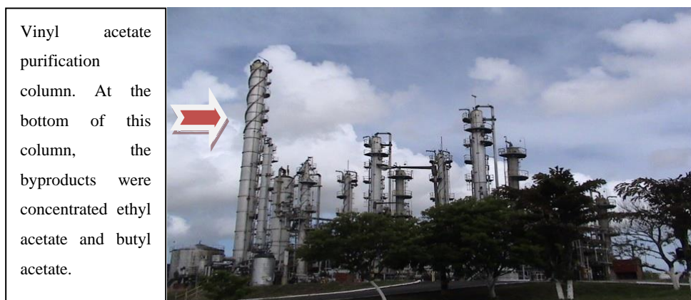
Fig. 2 ALCOOLQUIMICA's vinyl acetate unit. Photograph courtesy of Carlos Abdenor Neiva Nunes.
