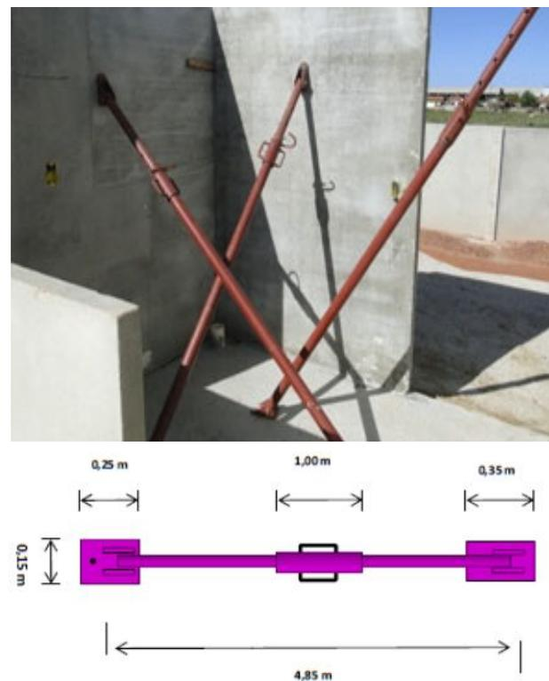
Fig. 2 Shoring and panel locking.
