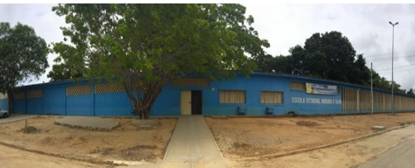
Fig. 2 Cobogós and brises elements on the façade of the State School Moreira e Silva.
