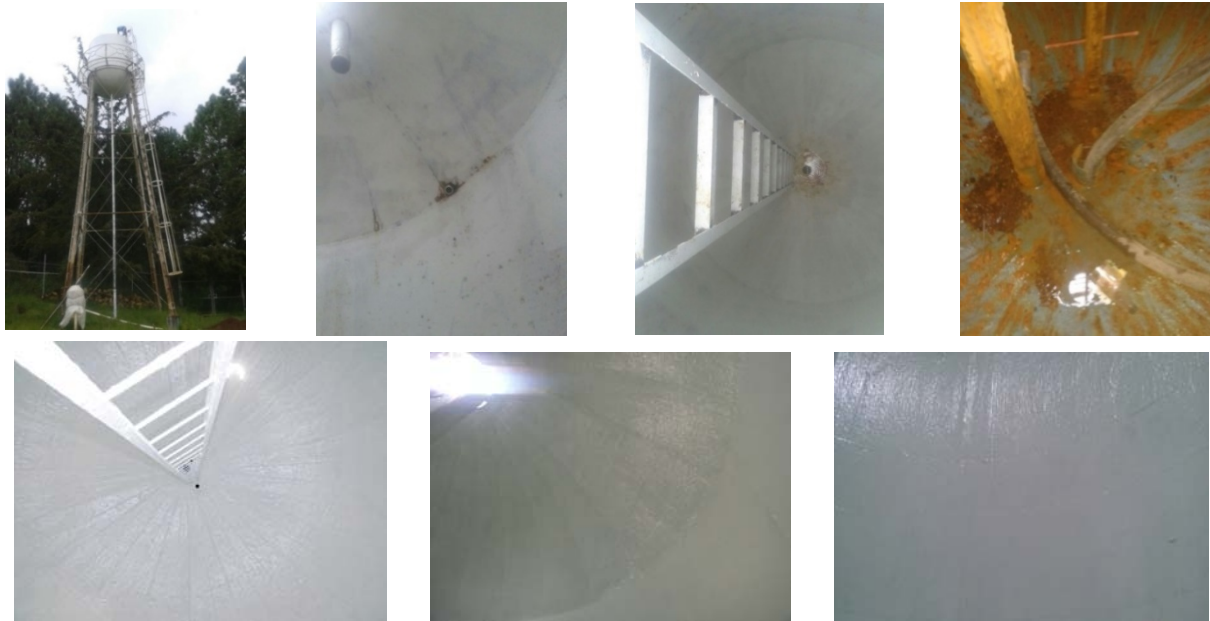
Fig. 3 Rehabilitation of metallic tanks with VITROACERO® (Concluded work).
