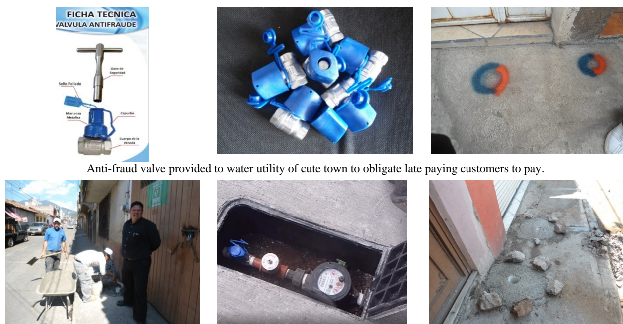
Fig. 5 Provision of multi-closing, anti-fraud valves, installed by water utilities (concluded work).
