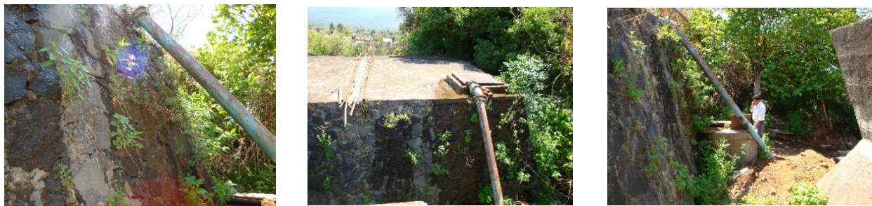
Tank with multiple fissures responsible for potable water waste
