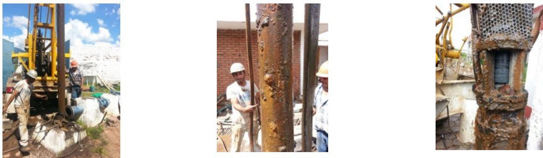
Extraction of pumping equipment in well number one in Quiroga to introduce video-inspection camera.
