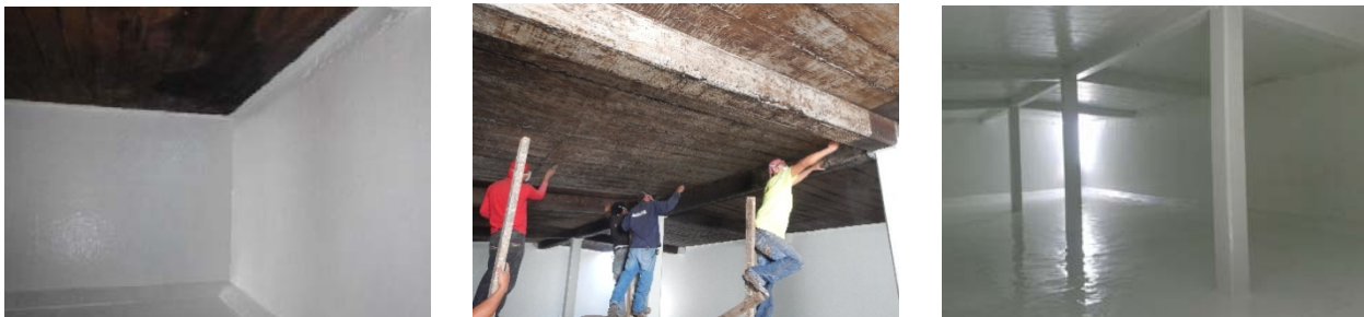
Rehabilitation Works to prevent the leak of water in The Superficial tank in Erongarícuaro, Michoacán, México.
