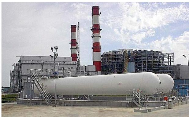
Fig. 1 Anhydrous ammonia storage tanks.
