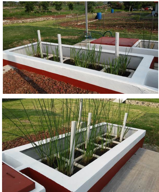
Fig. 1 Distribution systems and aeration pipes.
