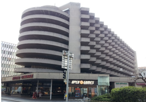
Fig. 1 Balestra multi-story car park in Lugano (photograph: A. Ruch).
