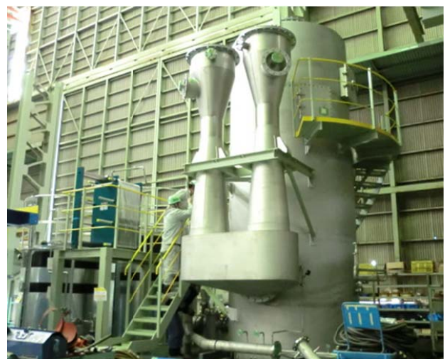
Fig. 5 IGS type wet scrubber (Photo taken during construction).
