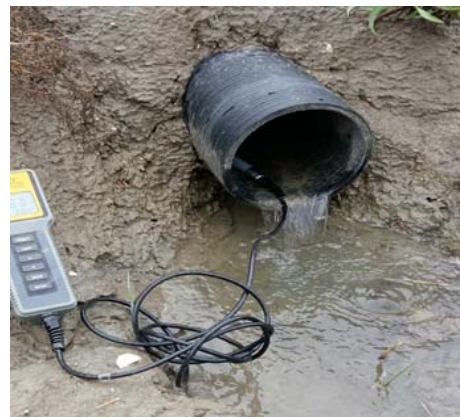
(b) drainage status of culvert drain
