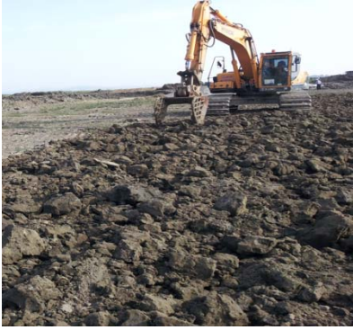
Fig. 6 Subsoil breaking using a backhoe.
