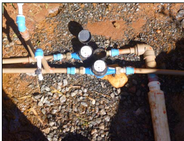
Fig. 4 Water Meters Used for Measuring the Net Volume of the Cells Output
